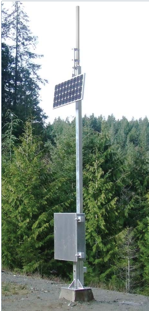
Mast Enclosure with solar panel and antenna.
