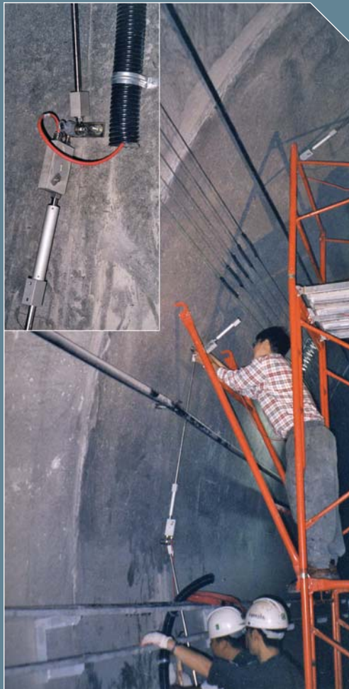
Typical installation of the RST Tunnel Profile System, with the inset photo showing a close-up of the final setup.
