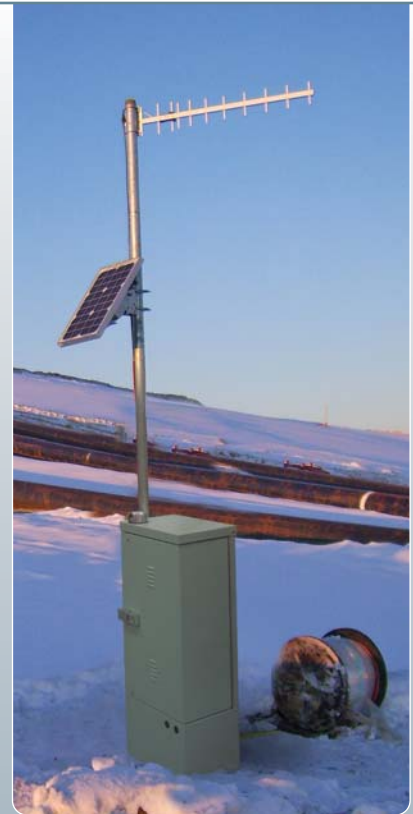
A typical L900 pedestal enclosure with solar panel. RST specializes in custom setups, contact RST for more details.
